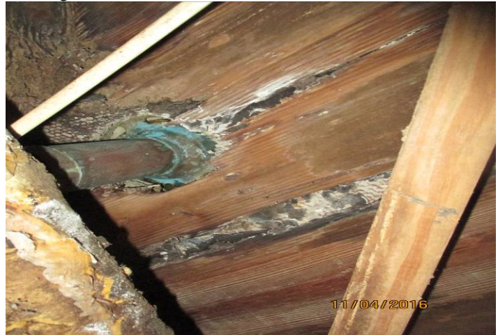
Master bath water damage
