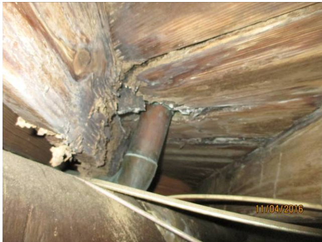
Master bath water damage
