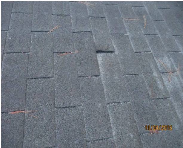
Water damage from leak over utility room
