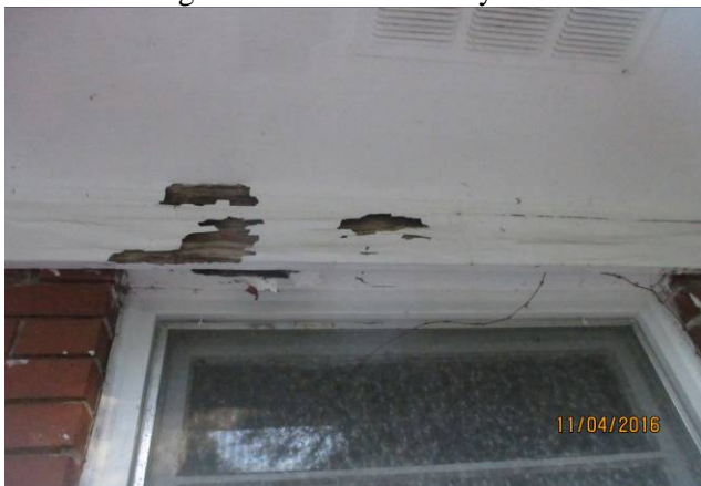
Water damage from leak over utility room
