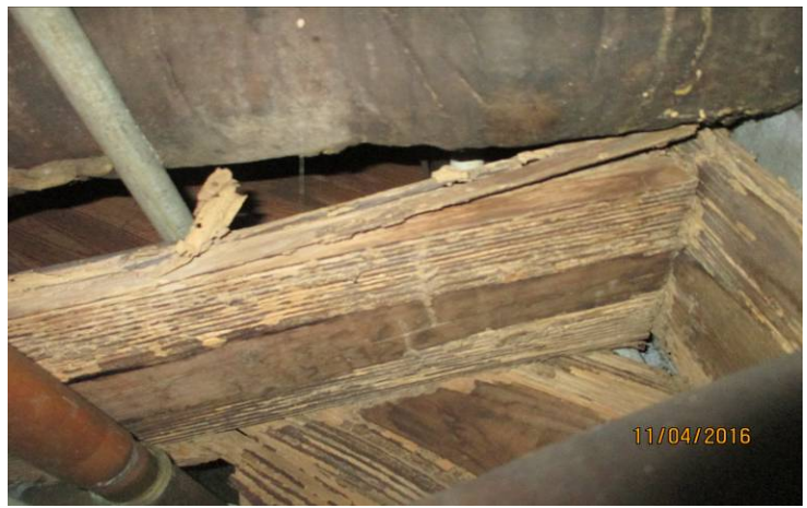
Master bath water damage
