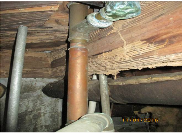
Master bath water damage
